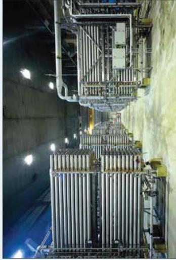
13 stages of PCI 3.6 m long B1 modules. A total membrane area of 4650m<sup>2</sup>.
